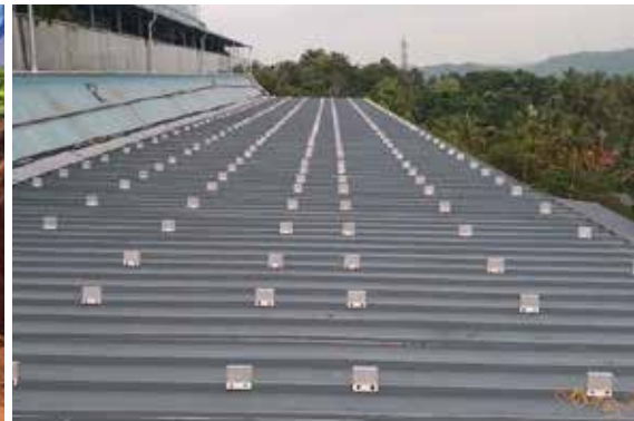
SITC of 300kWp solar photovoltaic system
