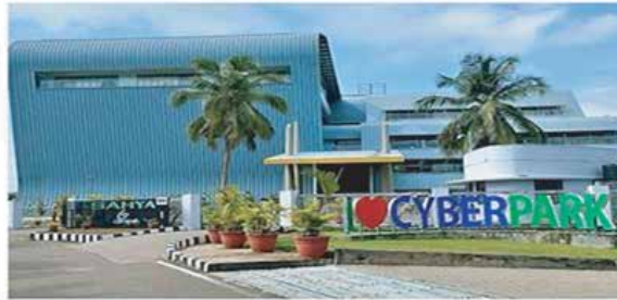
Proving its mettle: The seven-storey Sahya building on the 42.5 acres of the Cyberpark is fully occupied. FILE PHOTO
