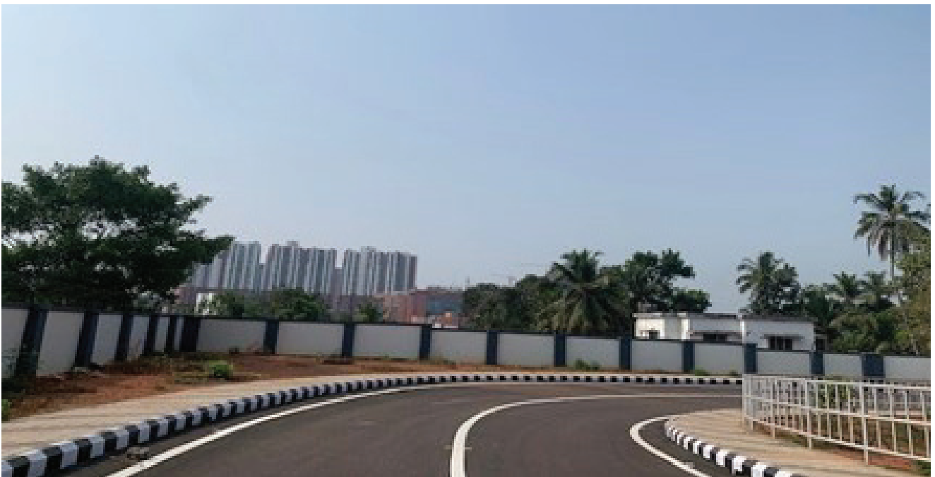
Compound Wall at Cyberpark
