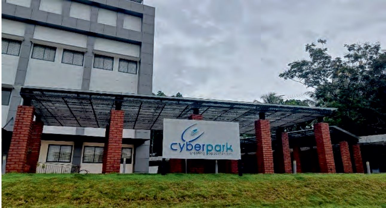
Construction of covered car parking and rest room at Park Centre
