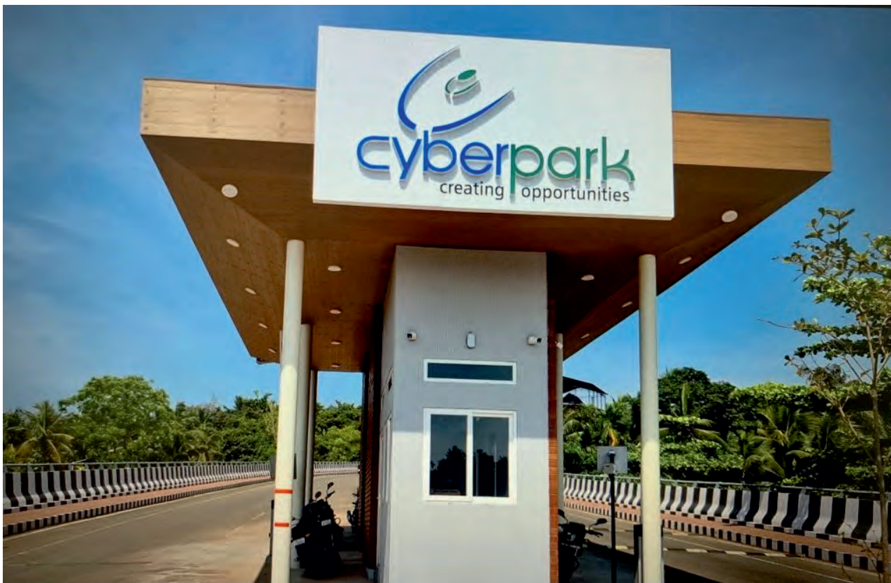
Construction of main entrance gate house at Cyberpark
