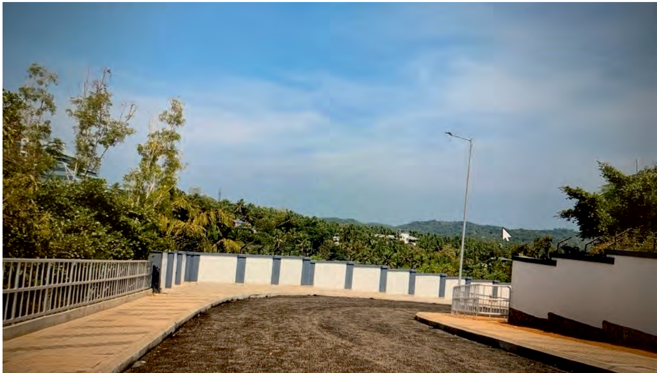
Construction of proposed road to non SEZ land parcels
