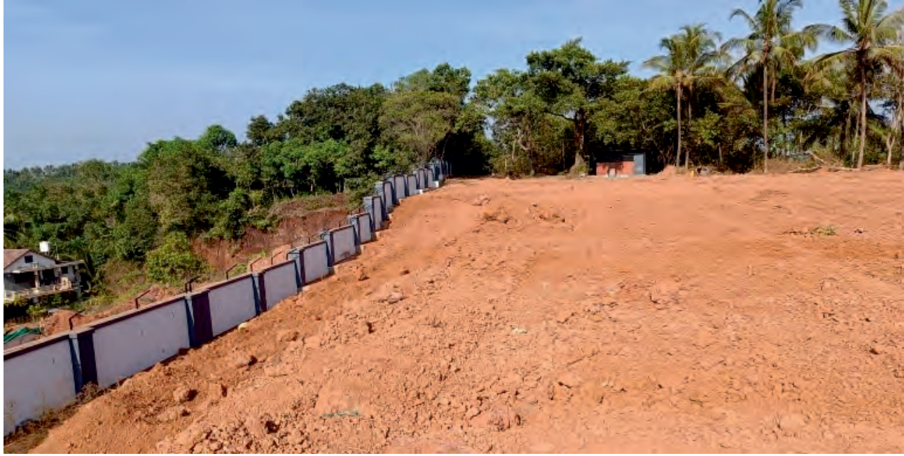
Compound wall at Cyberpark
