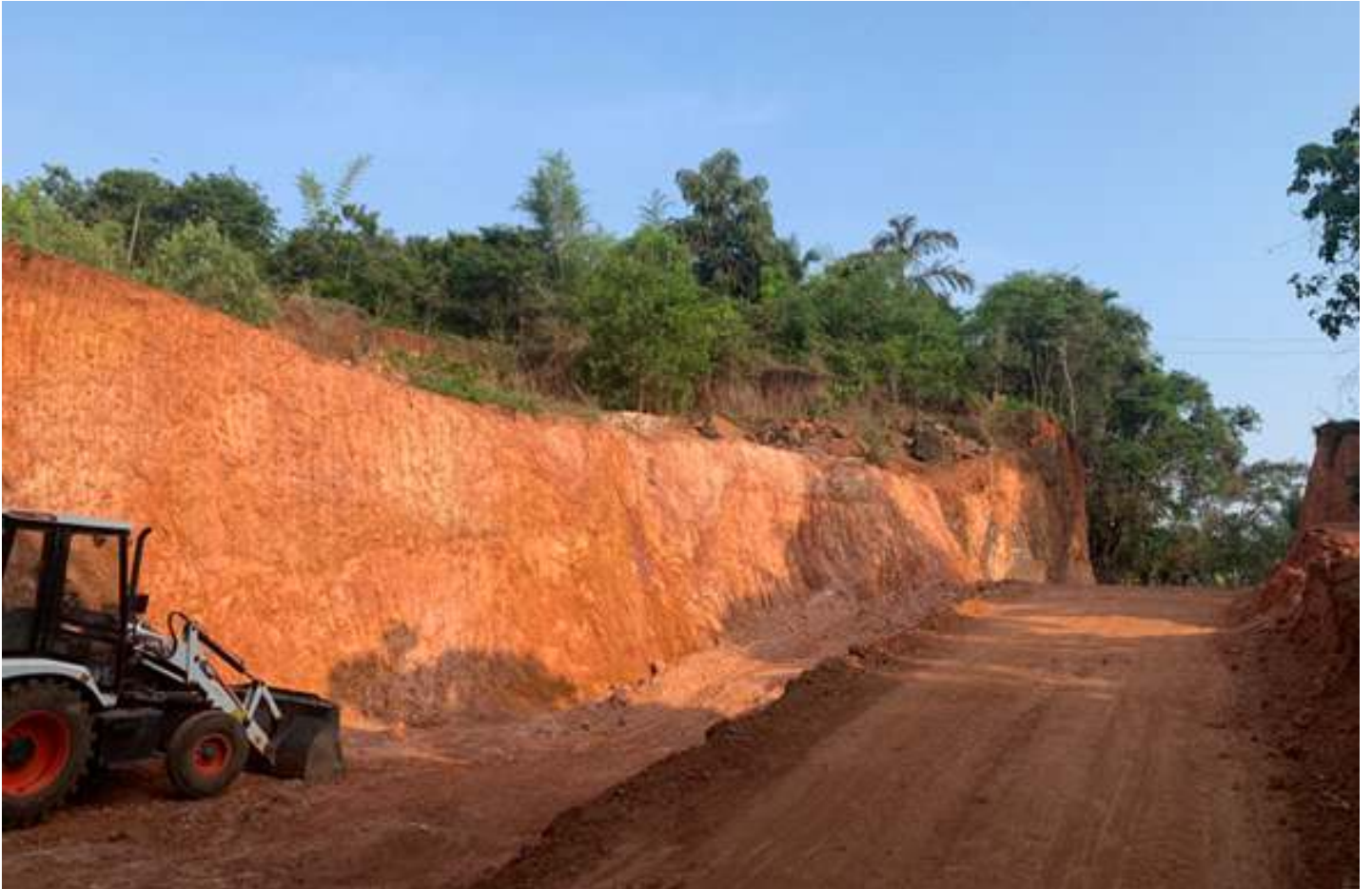
Road works to commercial plots at Cyberpark -work initiated
