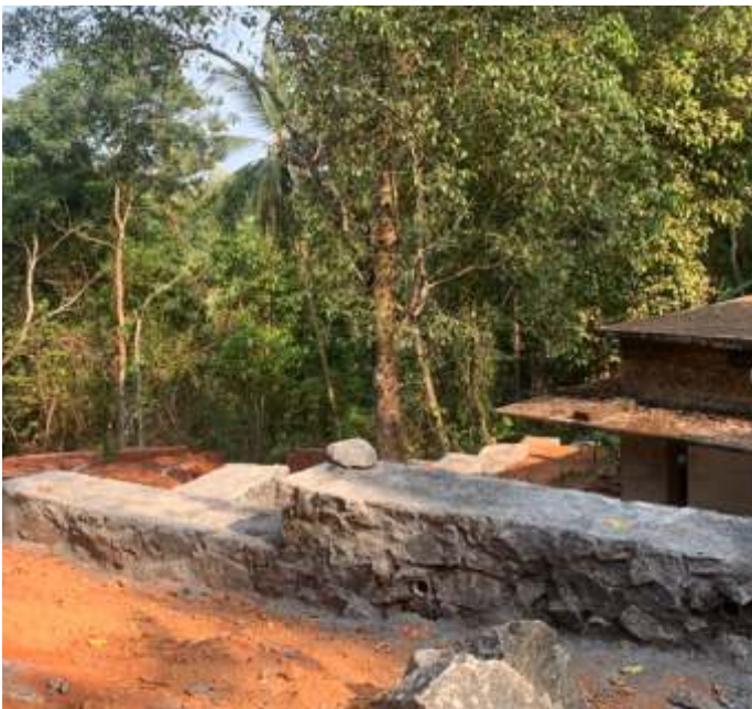
Compound wall work at Cyberpark
