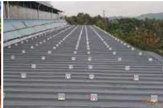
SITC of 300kWp solar photovoltaic system
