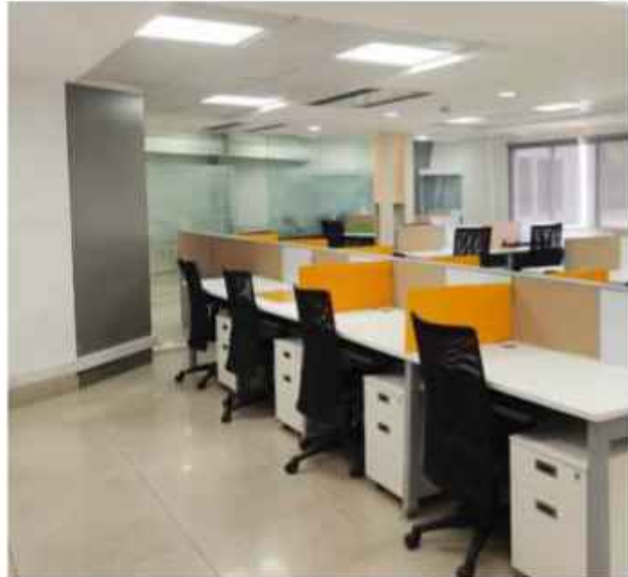
Renovation works of Incubation Hub
