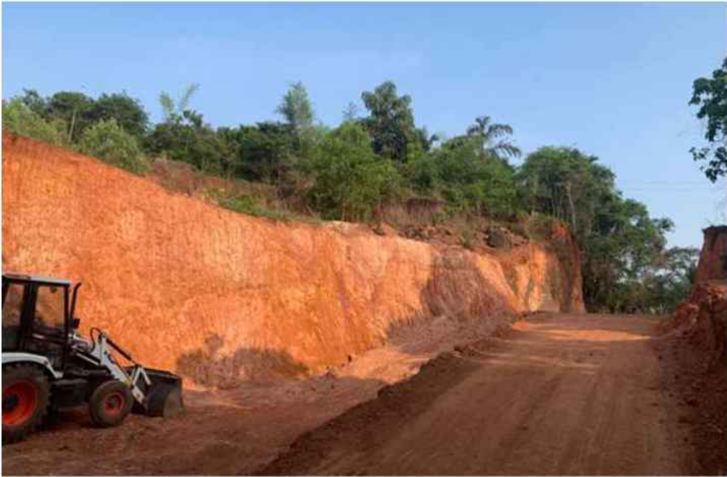
Road works to commercial plots at Cyberpark -work initiated
