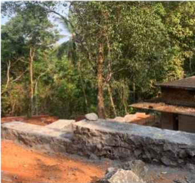
Compound wall work at Cyberpark
